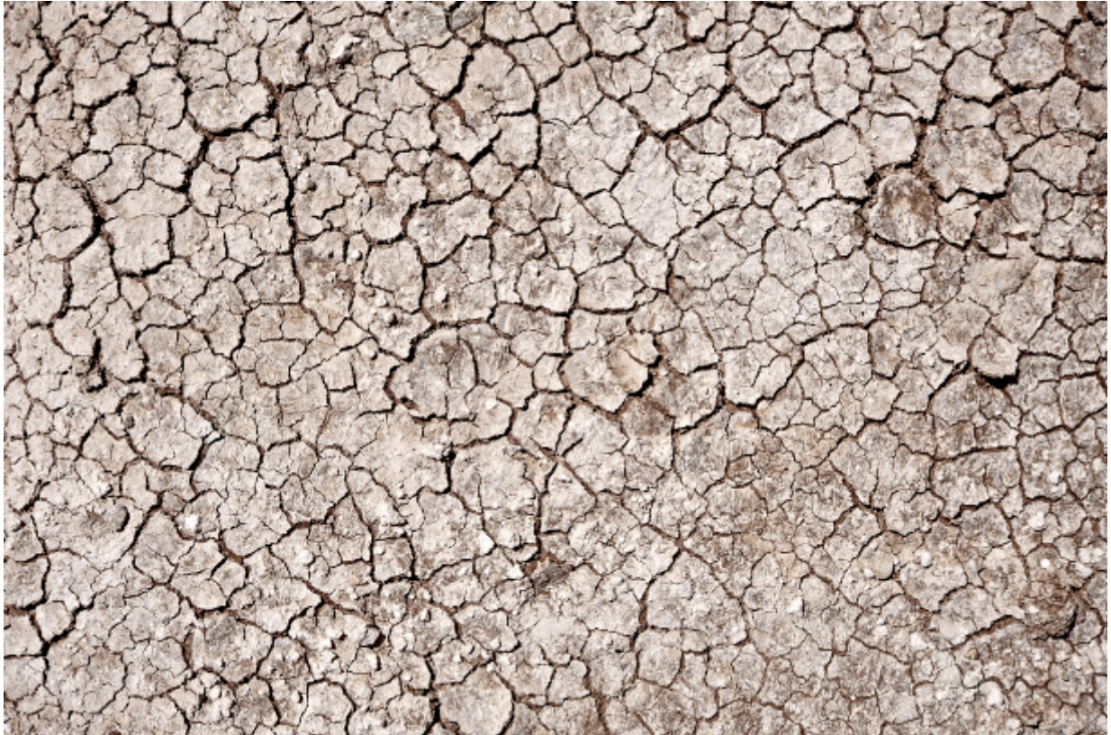
(a) Ground crack
